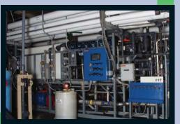
lean water is further purified by reverse osmosis. The water passes through a membrane which separates and removes any remaining solids. The purified water is cleaner
